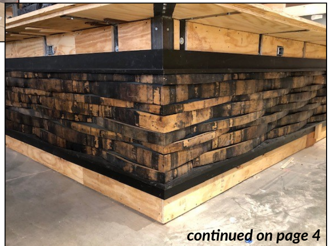
[above] East stairs and ramp for access to lower ballroom area. [left] New U-shaped bar, featuring a yellow accent wall, is taking shape! [below] Bar siding featuring restored whiskey barrel staves.
